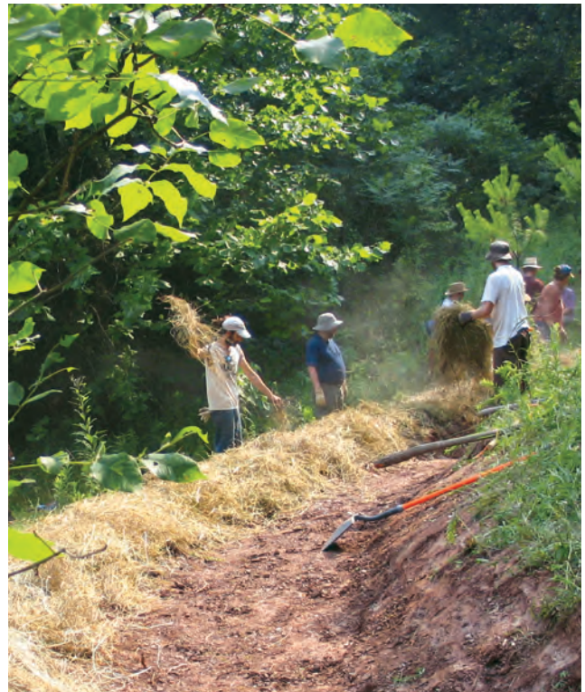
Mulching a newly constructed swale. Photo by Keith Johnson.
